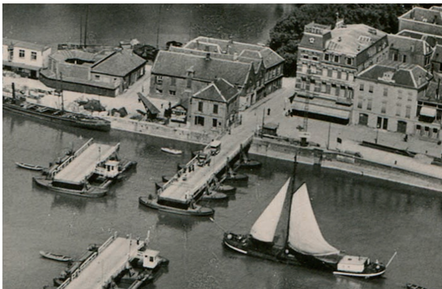
Point of interest 18: A pontoon bridge
