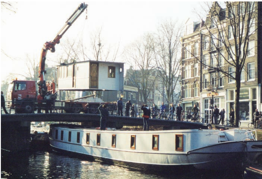
Point of interest 4: The pilothouse of Musard being dismantled
